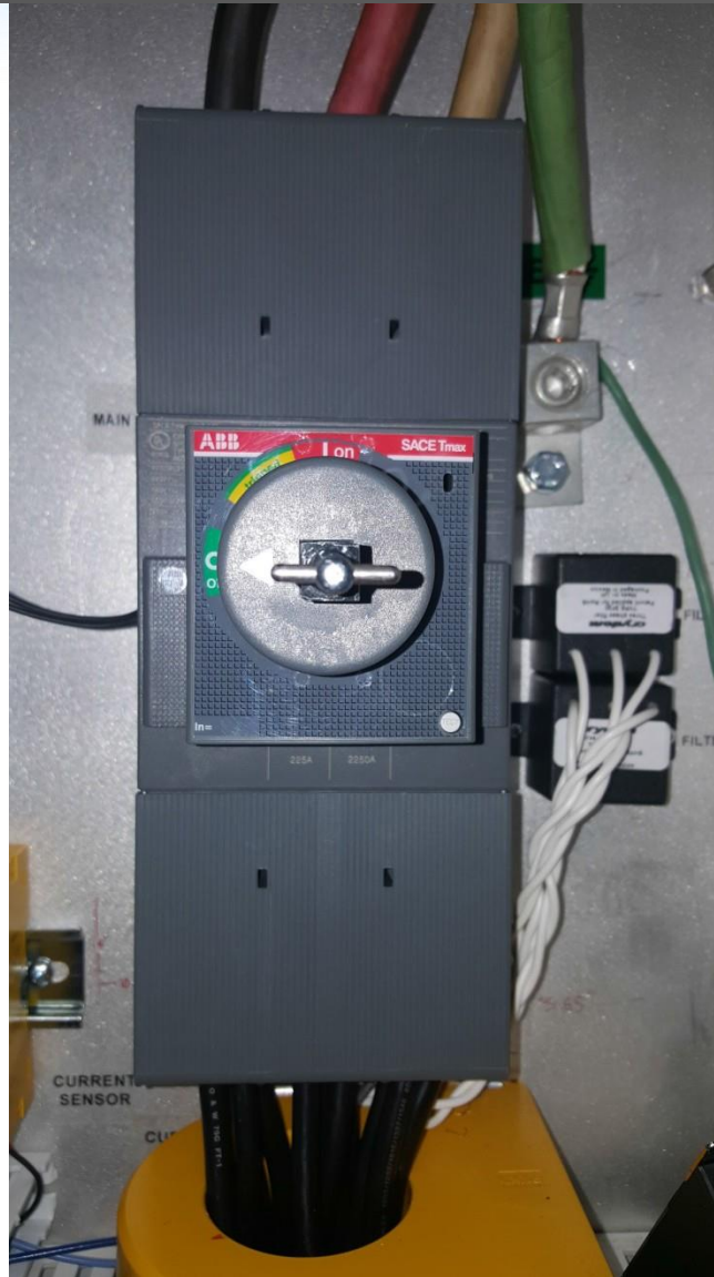
Figure 3-1: Main Circuit Breaker
